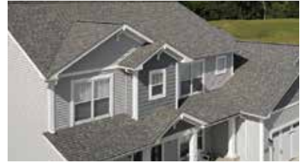
ROOFING AND VENTILATION
